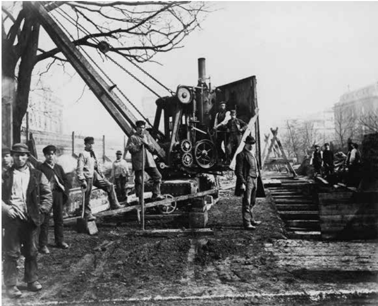
18. Henry Flather, A gang of workmen around a steam crane which is removing spoil from an excavation at Craven Hill , Bayswater Excavations, 1866-1868, © Museum of London.
